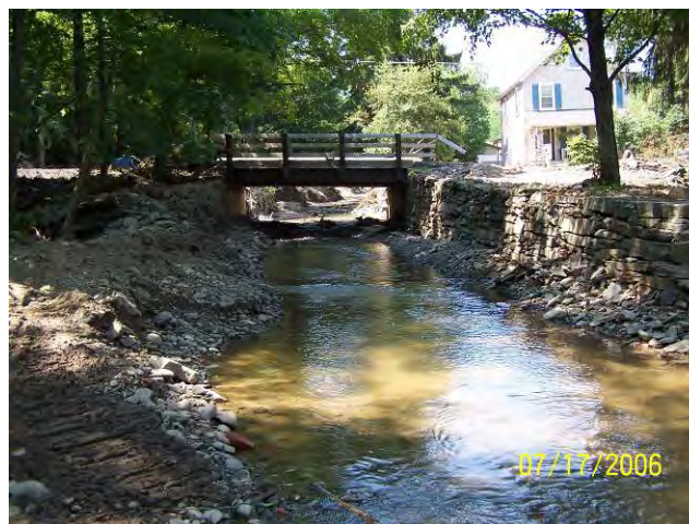
Figure 2.14 Bridge with no floodplain
