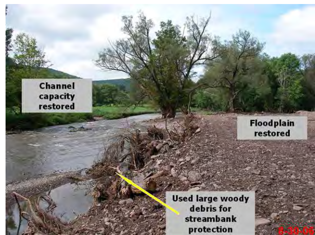
Figure 3.16 Stream construction using Regional Curve, typical cross-section and root wad.
