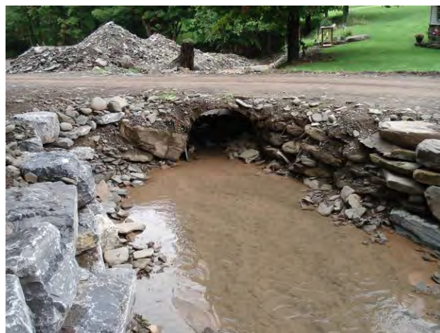
Figure 2.13 Culvert Conveying Holliday Brook
