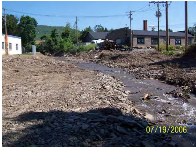
Figure 3.13 Shows stream channel after Post Flood Intervention.
