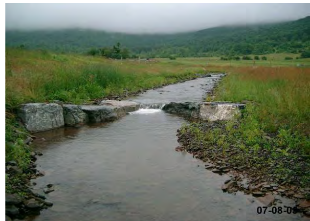
Figure 3.17 Rock Cross-Vane
