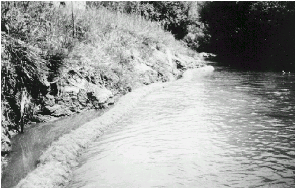
Figure 5.23a. Coir roll installed at stream edge (photo courtesy of Bestmann GmbH, Wedel, Germany)
