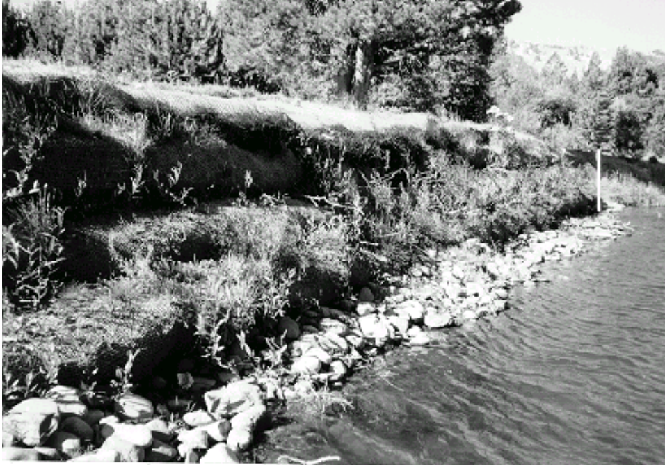
Figure 5.32. Upper Truckee River site after construction
