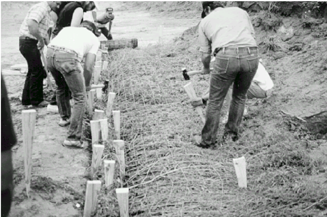
5.26c. Installing a brushmattress and wattling
