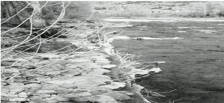
Figure 5.17. Installed log revetment
