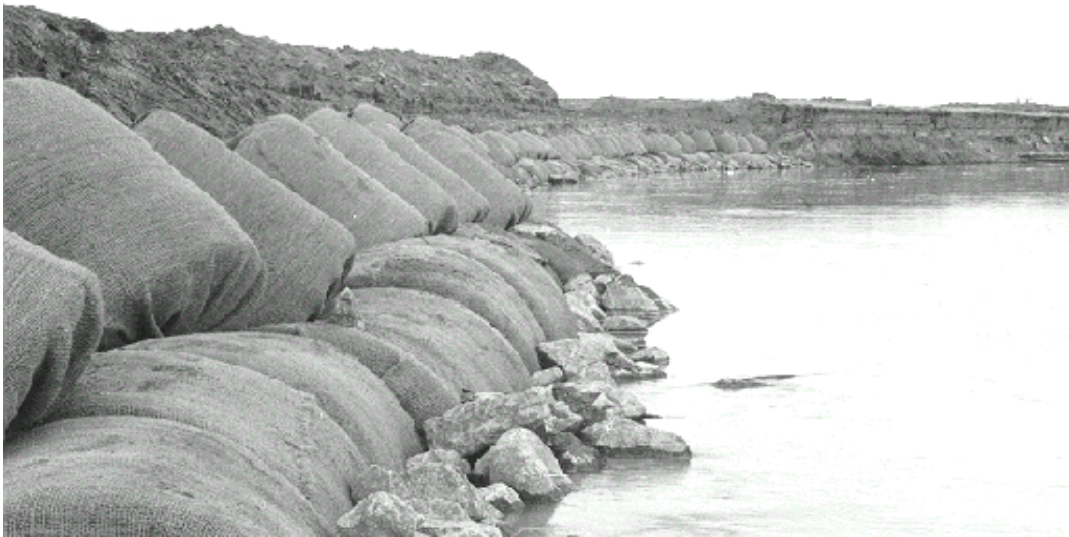
Figure 5.8. Rock toe with hay bale cylinders
