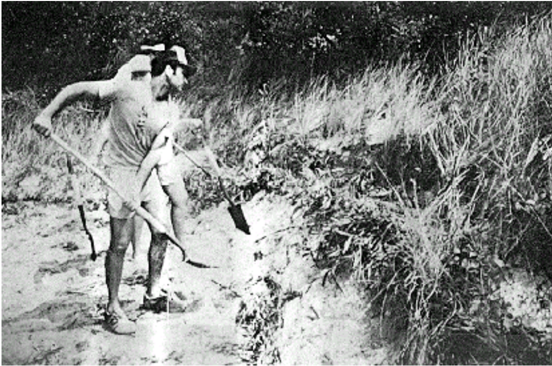
Figure 5.28. Covering brush layers immediately
