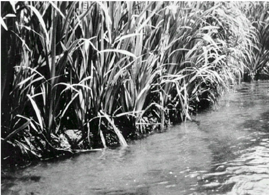
Figure 5.23c. Close-up of coir roll with vegetation (photo courtesy of Bestmann GmbH, Wedel, Germany)
