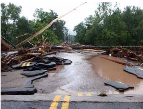
Left: Bridge Street Bridge in Phoenicia shortly after Hurricane Irene flood waters began to recede. Notice how much the double yellow line moved because of the force of the flood waters
